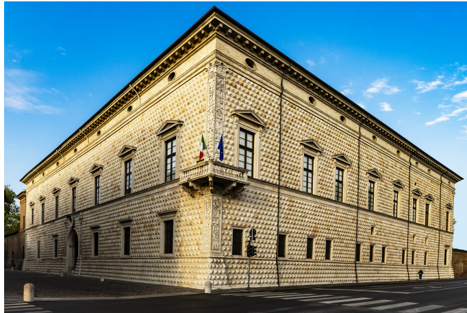
Diamonte Facade Highly Commended Eric Brandseth
