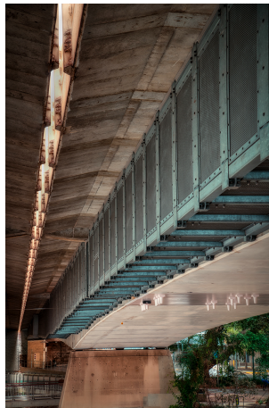
Goodwill Bridge Commended Greg Suter
