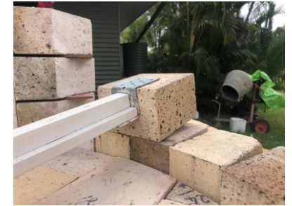
Work in Progress 0985 Accepted Col Pieper
